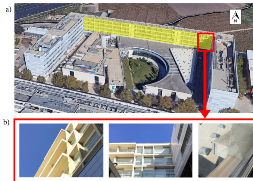
Figure 5. Faculty of Fine Arts at Universitat Politècnica de València. a) South façade, highlighted in yellow, indicates the area for the implementation of the photovoltaic cantilever. b) Structural constraints along the rows
