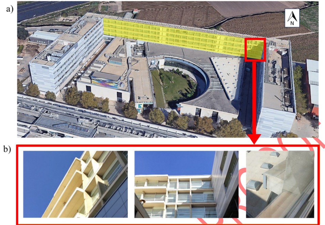
Fig. 5 Faculty of Fine Arts at Universitat Politècnica de València. a) South façade, highlighted in yellow, indicates the area for the implementation of the photovoltaic cantilever. b) Structural constraints along the rows
