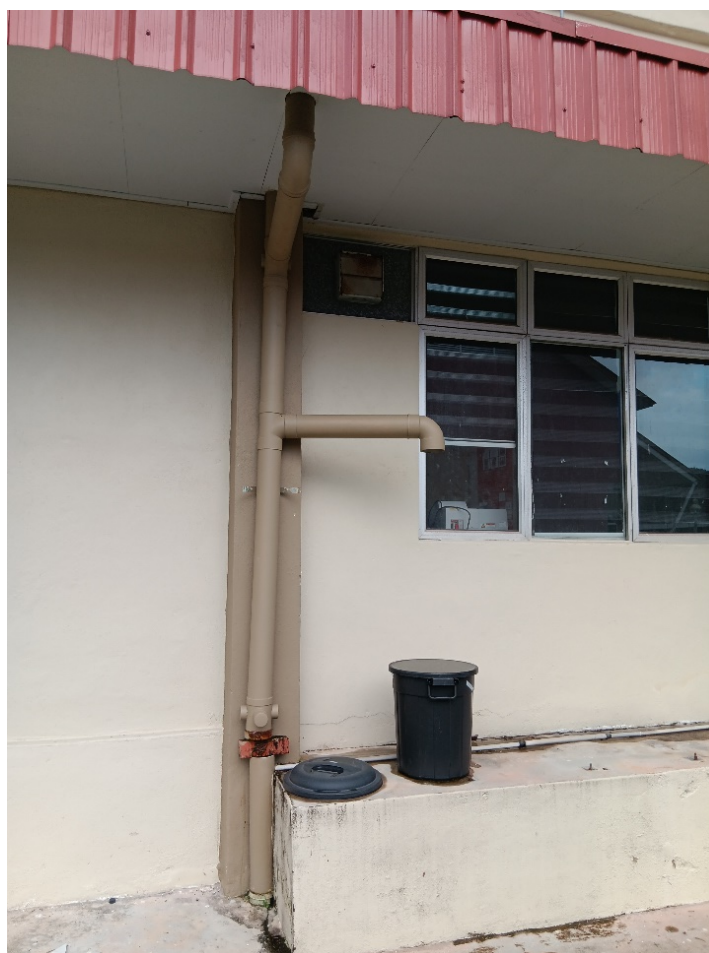
Figure 2. Rainwater harvesting system in the N12 building of UTM
