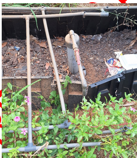
Figure 2. A plastic biogas dome installed underground but no longer functional due to lack of feed material and water
