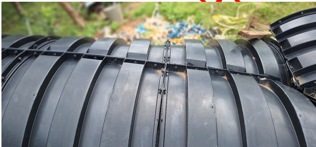
Figure 1. A plastic biogas dome material that was assembled onsite but has to be replaced soon because of poor workmanship and deterioration of the material due to exposure to sun
