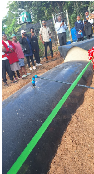
Figure 3. Inflatable fixed biogas dome recently constructed by STREEC and inaugurated by the Eswatini Ministry of Natural Resources and Energy
